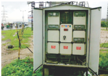
Electric Control Panel Installation for BRTS
