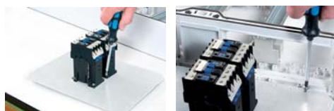
Device installation on mounting plates
