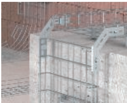
Complete installation Illustration of complete C mesh cable tray mounting.
