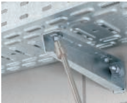
Quick fastening of cable tray on the bracket The quick fastening is pushed upwards and turned through 90°. After locking, the quick fastening is fastened permanently by tightening it.
