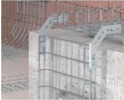
Stand-off with vertical bend application Installation of a vertical bend using installation profiles, type MW, for stood-off C mesh cable trays.
