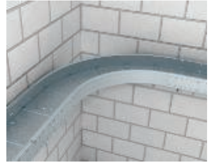
Installation of 90° bend Bend in combination with wide span cable trays. The bend is connected to the wide span cable tray using external connectors and a joint plate.
