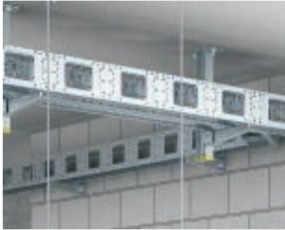
BKK system application Installation of the BKK system under the ceiling using IS 8 supports.
