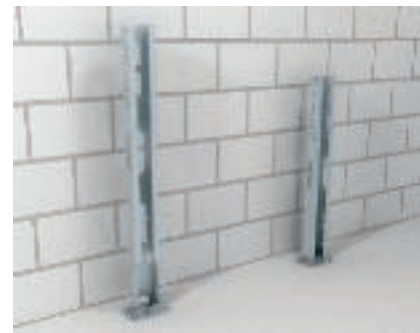
Installation of motor connection column with column foot Fastening of the motor connection column, type MAS 140/10, to the floor using column foot, type SF 140/11.
