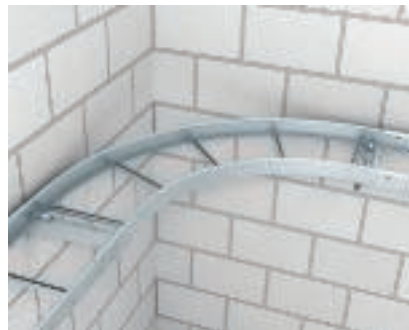
Installation of a cable ladder bend Connection of the cable ladder with the bend, type LBI 90. Additional supports should be planned for the area of the fittings.
