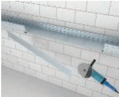
Creation of a tee with add-on corner Removal of the side rail from the ongoing wide span tray.
