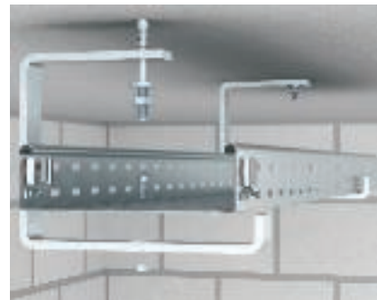
Direct fastening of the ceiling bracket Direct mounting of the AHB ceiling bracket with anchor bolt on the ceiling. Maximum cable tray width 400 mm.
