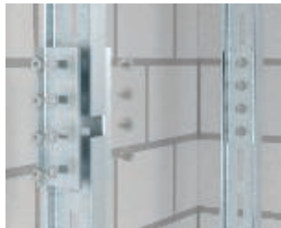
I support connection Installation of the I support connector VIS 8 to connect IS 8 supports.
