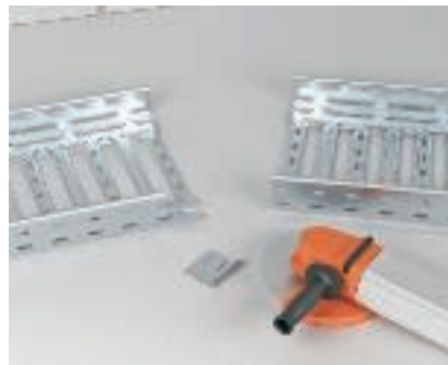
Horizontal angle connection of cable trays Step 1: After specifying the required angle, the side rail is cut off on one side.
