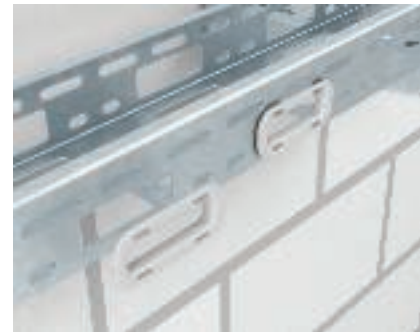
Side rail cable protection ring Insertion of the cable protection rings, type KSR-DR 910, in the side rail of the AZ channel.
