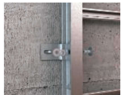
Fastening of industrial vertical ladder Industrial vertical ladders are fastened to steel girders using mounting angle, type BW80/55.
