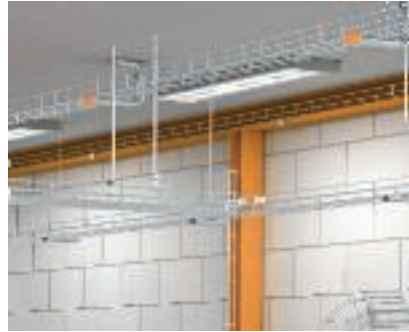
View of a complete installation Illustration of complete mesh cable tray mounting.
