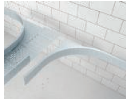
Creation of a tee with add-on corner Installation of the second add-on corner, type WEAS 110.
