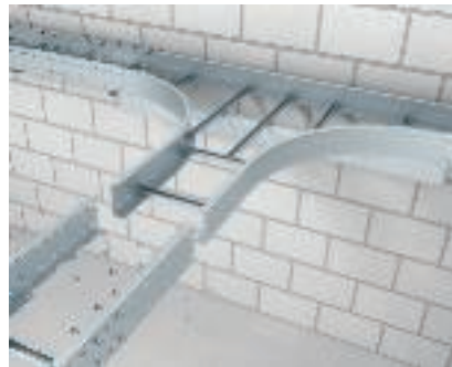
Installation of tee Tee in conjunction with wide span cable ladder. The tee is connected to the wide span cable ladder using external connectors.
