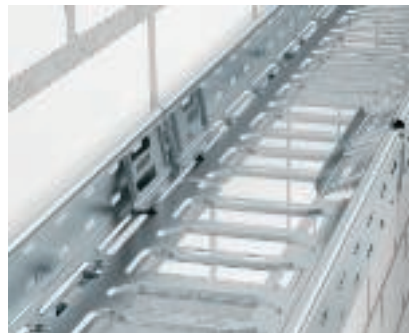
Mounting of Magic KTSMV straight connector set Simply clamp the two side sections of the connector set in the side rail.
