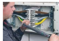
The terminals need to be tightened with the appropriate torque
