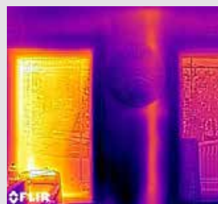
Warm Drain Pipe in Wall
