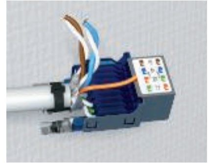
Device connection – cable sorting Attach the individual wires according to the connection table and fix them using the contacting terminal.
