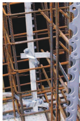
Fig 7 : Interconnection of reinforcement to be used as down conductor
