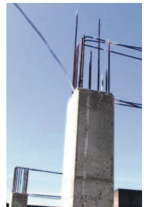
Fig 7 : Interconnection of reinforcement to be used as down conductor
