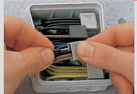
Connection: Insert stripped solid conductor FULLY
