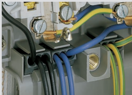
Push-wire connectors used in a cable duct with double power outlet
