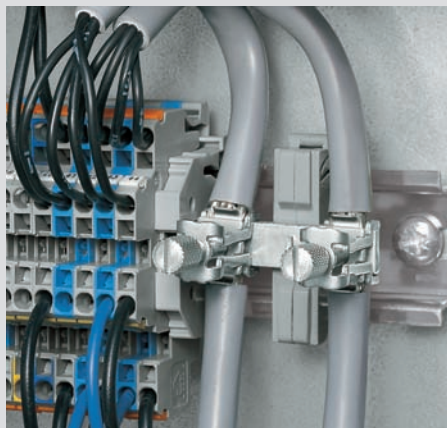
– carrier with grounding foot, busbar parallel to the rail
