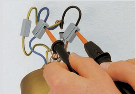
Testing through separate test slot
