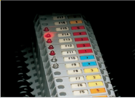
Blown fuse indication by LED or neon lamp
